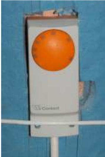
Setting the hot water thermostat to 50°C (see above) will result in hot water and will be very economical to run. However we recommend that the set-point is raised to 65°C for one hour each week to sterilise any bacteria that may colonise the hot water cylinder.
