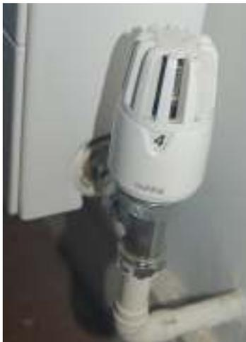
The radiator thermostat works by allowing heat into the radiator until **the room** heats to a specific valve.
